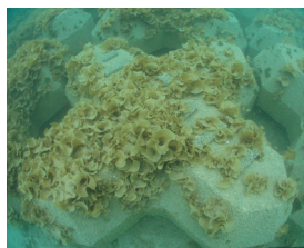
Marine plants thriving on tetrapods bonded with slow water-soluble glass.
