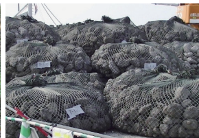
submerged breakwater structure (Filler: Iron and steel slag hydrated matrix)
