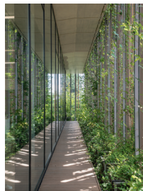
Solar radiation control by wall greening (Regional native climbing plant)
