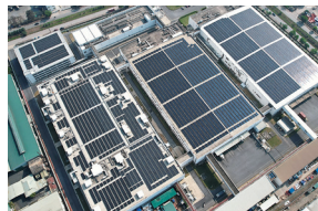
Installation of solar panels
