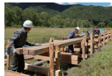
Installation of wooden walkways
