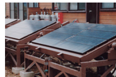
Solar panels installed in mountain huts
