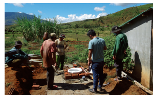
Toilet construction workshop in Vietnam (Foundation for International Development / Relief)
